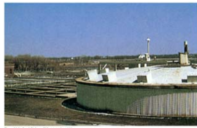
Figure 20.48: Aeration tank showing the activated sludge process. © 2004 Pearson Education, Inc.
